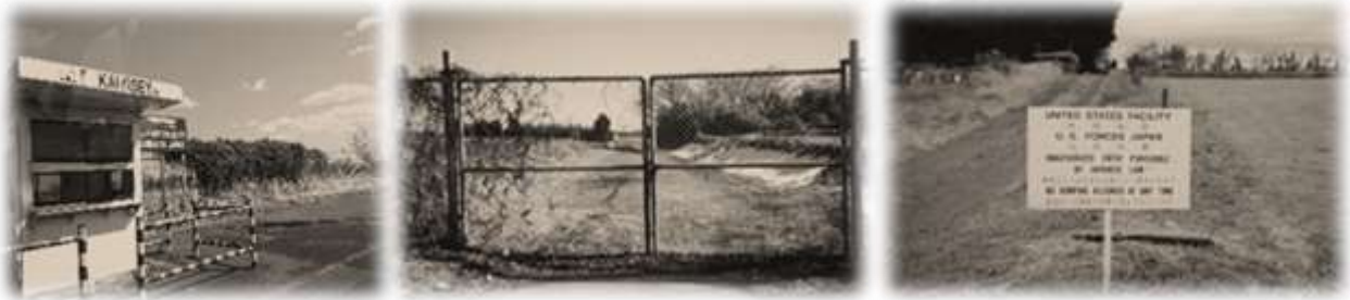
The land was surrounded by fences
